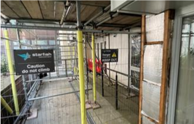
A photo showing Phase 2 North Elevation – Existing cladding removal works commenced
