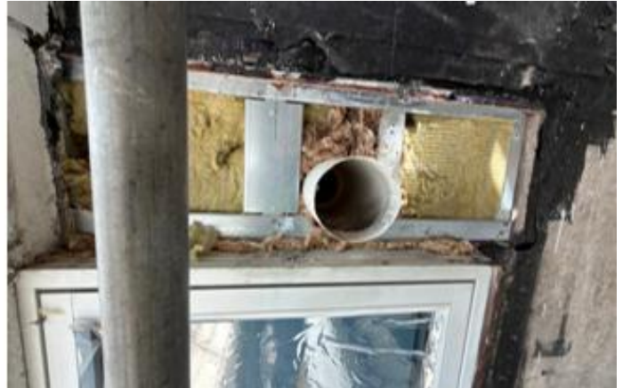
A photo showing Phase 1 South Elevation – Additional SFS studs installation to facilitate new s/s vent duct sleeves installation progressing
