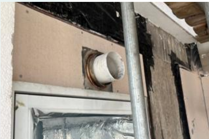
A photo showing Phase 1 South Elevation – New s/s vent duct sleeves installation commenced and progressing
