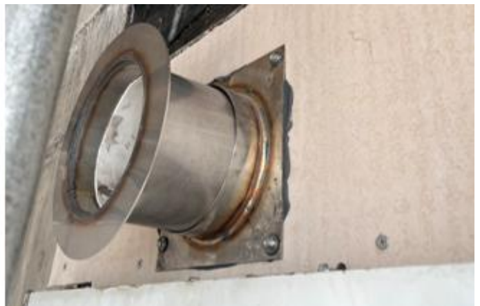
A photo showing Phase 1 South Elevation – New s/s vent duct sleeves installation commenced and progressing
